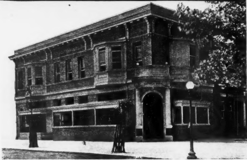
(ABOVE) PROPOSED COLORED Y. M. C. A. BUILDING AT ST. LOUIS, MO., BEING ERECTED AT A COST OF $180,000
